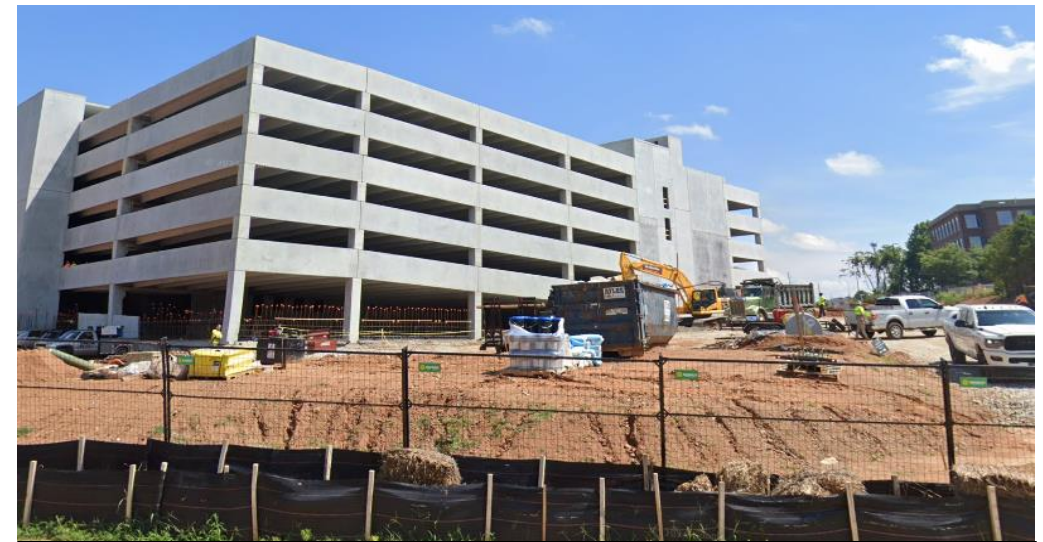
Kensington Station TOD Construction
