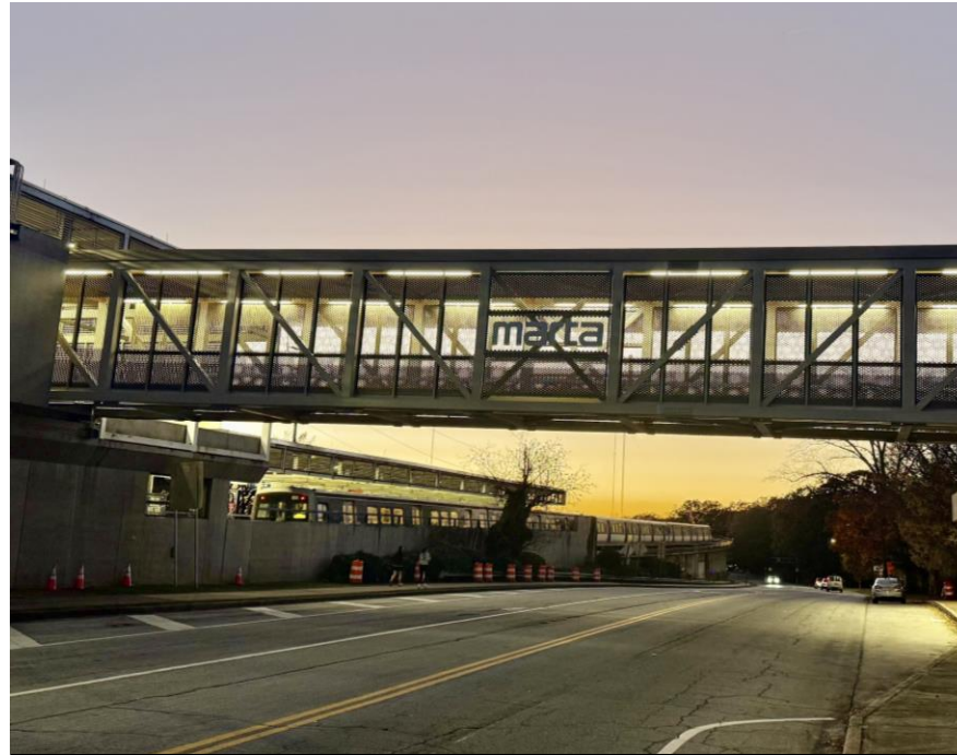
New North pedestrian bridge
